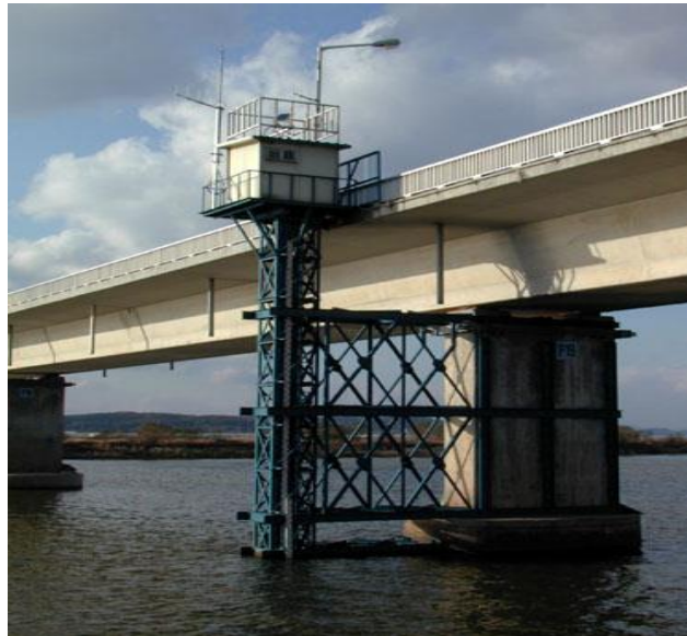
Fig. 4-2 Float gauge (with stilling well)
